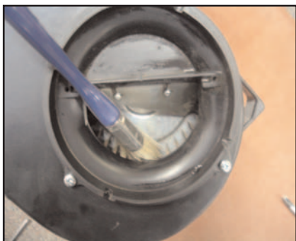
Open access door. Remove 2 screws.
