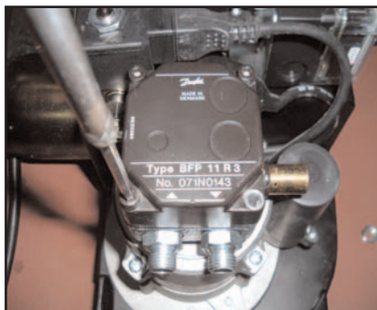
Check and clean pump filter.
